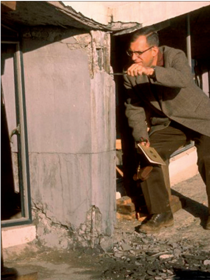
Ray Clough at the Lorenzas Arenas Market, Concepcion, Chile, 1960 Chile Earthquake.
